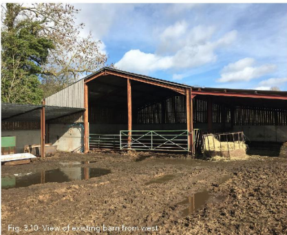
Fig. 3.10 View of existing barn from west
