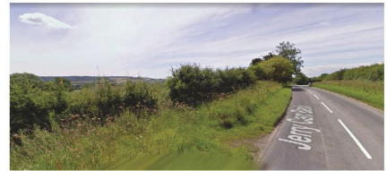
Fig. 5.2: Existing secondary field access gate from Jerry Carr Bank (looking west)
